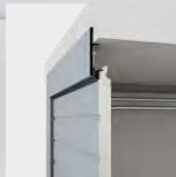
In Front Of The Lintel
